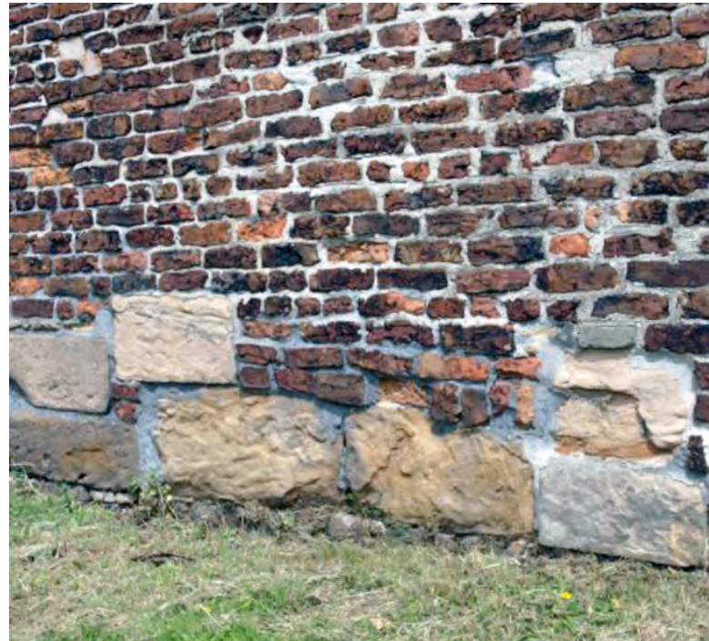
Original sandstone foundations of present-day barn
